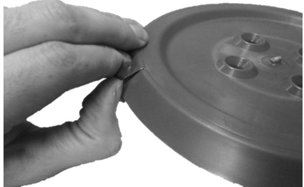
9. After the concrete is poured, remove the outer rim of the protective cover. You can now finish the pool surface.
