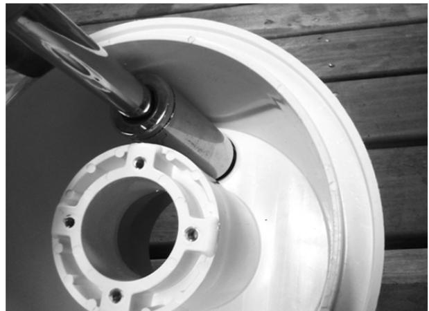
3. Insert the cable gland into the threaded socket on the conduit adaptor, ensure the rubber washer is on the thread of the cable gland. Tighten with a socket wrench.
