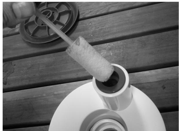
5. Apply PVC solvent primer to the conduit adaptor and to the conduit. Allow to rest for one minute, then apply PVC solvent cement (non-pressure type N is sufficient) to both parts.
