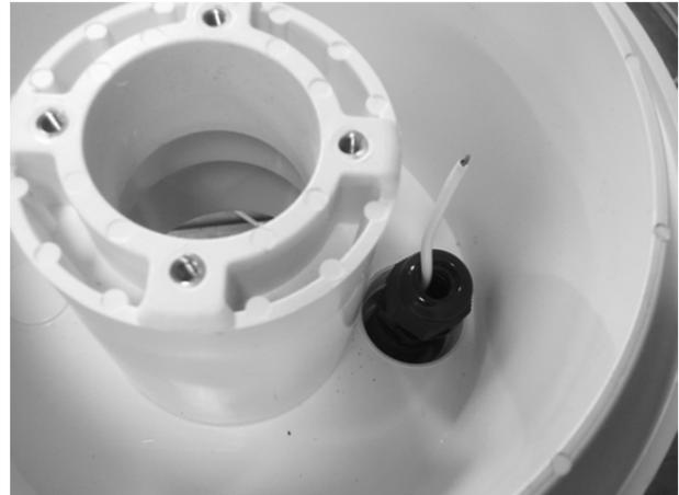
4. Thread a thin piece of cord or tough string through the cable conduit from the beginning of the conduit (near the transformer) all the way through to the light niche. This will be used to pull the light's power cable through later on. We recommend using sweeping bends and not elbows, to make it easier to pull the cable through.
