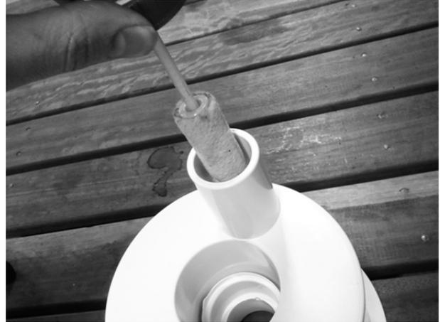
1. Apply PVC solvent primer to the conduit adaptor and to the socket on the niche. Allow to rest for one minute, then apply PVC solvent cement (non-pressure type N is sufficient) to both parts.
