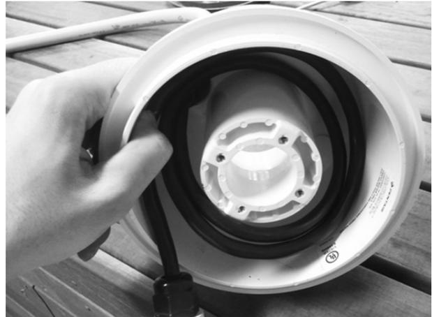
11. Pull the power cable through, leaving about 1m of cable to allow inspection of light above water surface.
