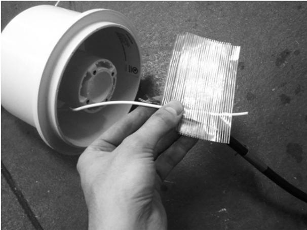
10. After the surface is finished. Remove the protective cover. Tape the end of the light power cable to the cord or rope that was threaded through the niche. Make sure it is secure and won't pull apart when tugged.
